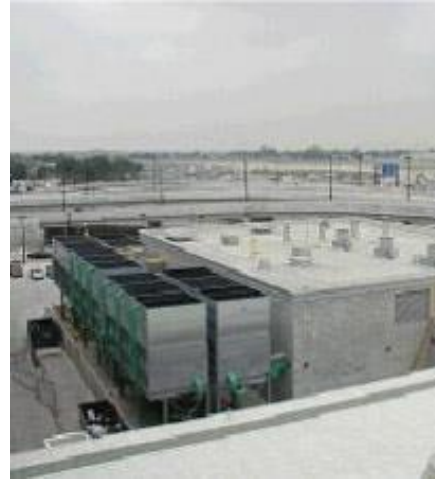
Midway Airport, Chicago 14,000 ton-hours – 49,4 MWh 528,988 kg ice [14]
