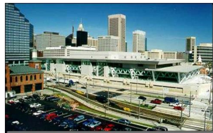
Baltimore Convection Centre 89,665 ton-hours – 317 MWh 1,853,537 kg ice [14]
